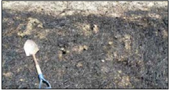
Figure 6-2. Typical California ground squirrel burrows on water-side slope of a clayey levee. (Department of Civil and Environmental Engineering, University of California, Berkeley, CA.)
