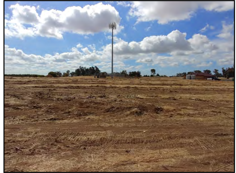
View of the cell phone tower and associated structure within the central western portion of the Project Area. Photo taken October 20, 2017.
