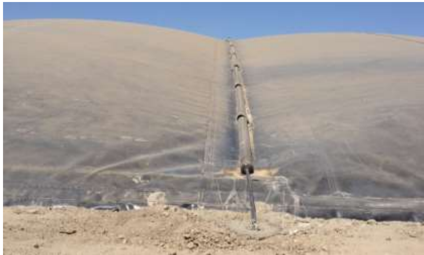
Figure 1: Covered Lagoon/Pond Digester
