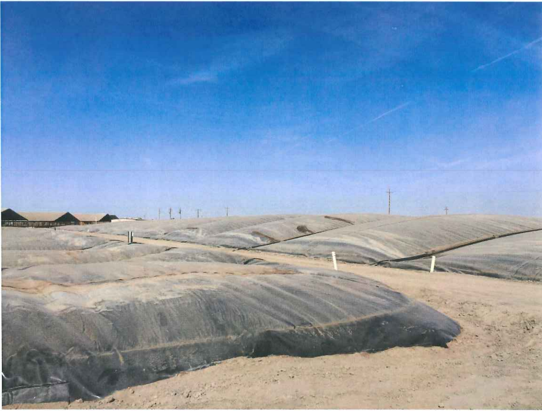
Figure 3: Example photo of lagoon digester vessels
