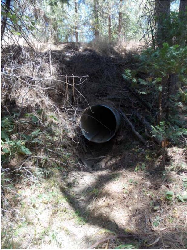
**Photograph 11 - Existing 30" Culvert Outlet**
