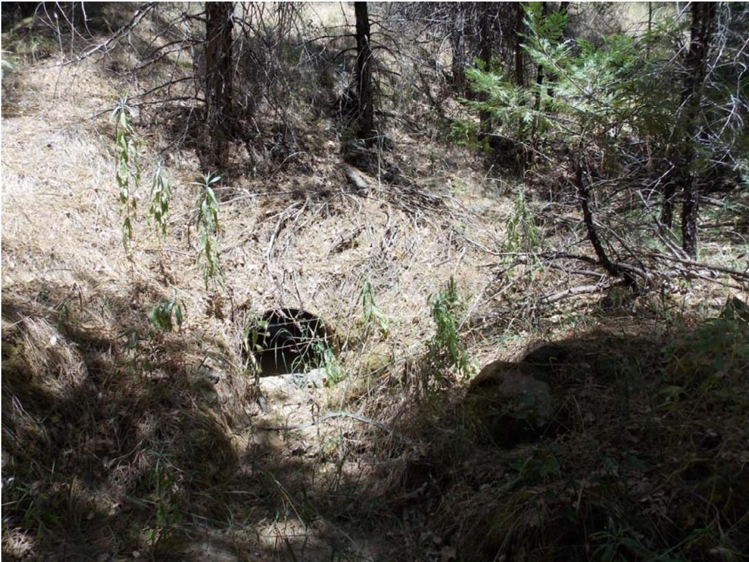
**Photograph 10 - Existing 30" CMP Culvert Inlet**
