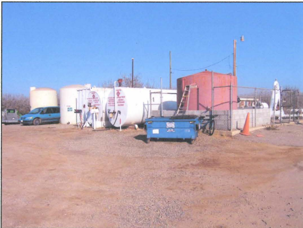
Figure 2d. Water pumping facility adjacent to packing shed on the east.
