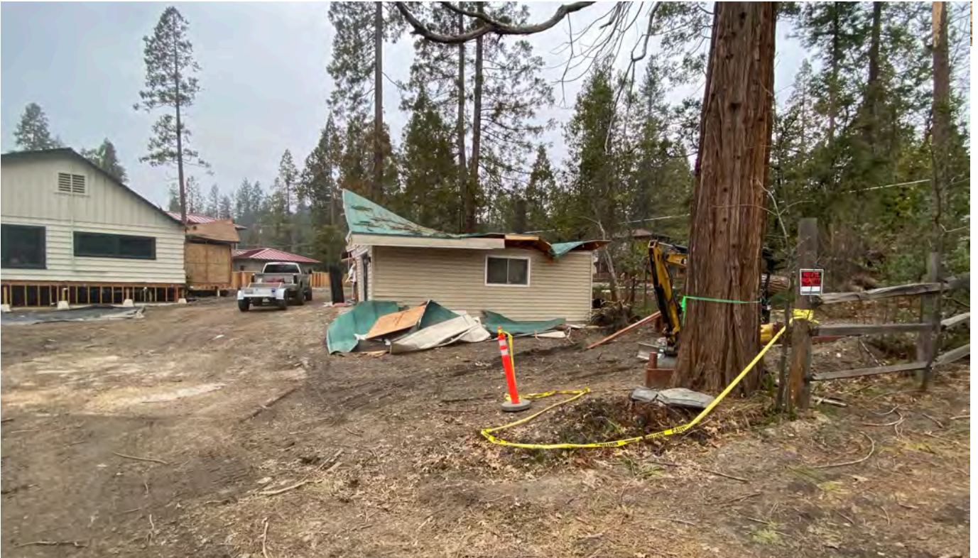
SITE VISIT PHOTOS FROM SOUTHERN PROPERTY LINE
