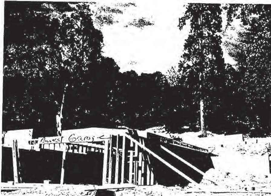
Guest garage prior to completion
