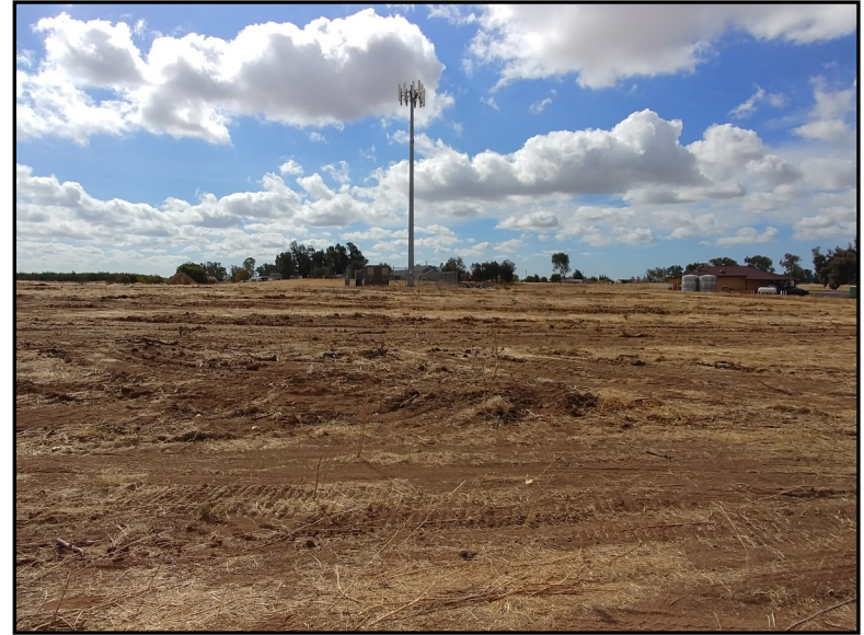
View of the cell phone tower and associated structure within the central western portion of the Project Area. Photo taken October 20, 2017.
